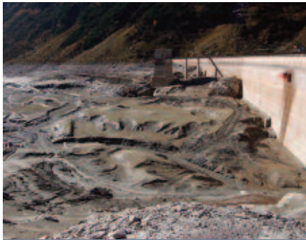
Figure 3. Sedimentation in an Austrian reservoir after a controlled reservoir level drawdown (courtesy: Gökler)
