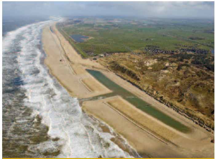
Figure 3. Aerial overview of the Hondsbossche Dunes
