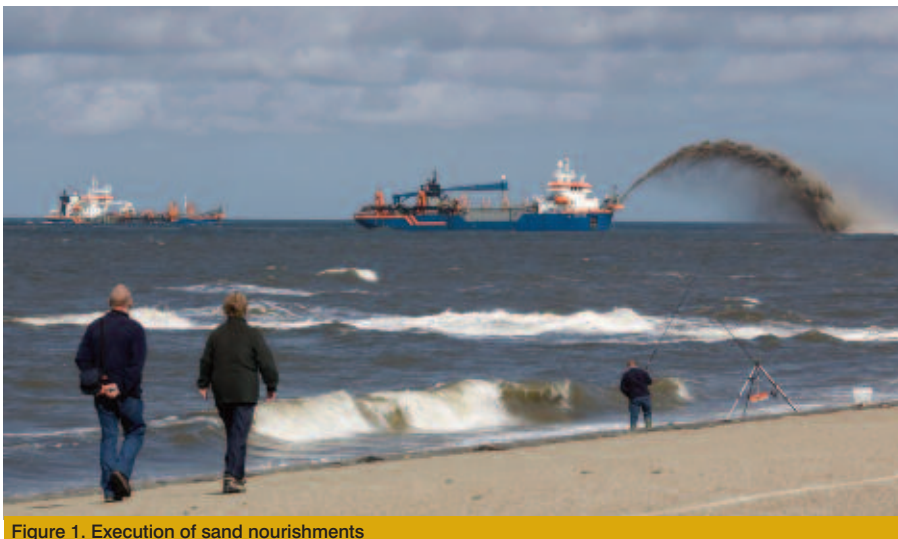
Figure 1. Execution of sand nourishments
