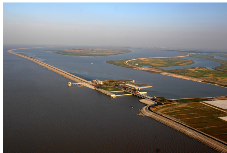
Figure 3. The upper water intake system.
