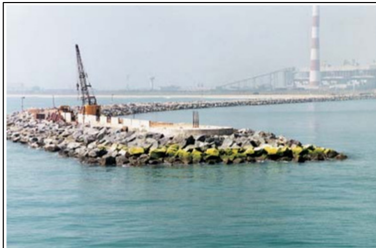
Figure 5. Breakwater constructed in New Ennore coal project ( http://www.ennoreport.gov.in/ ).
