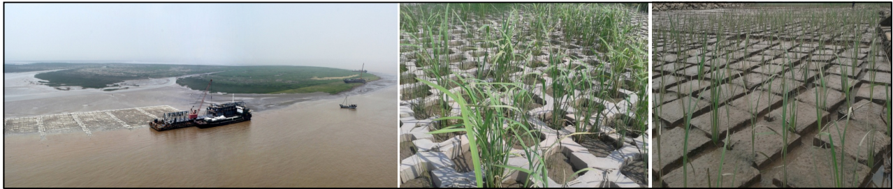
Figure 7. First stage renovation works of a waterway in Yangtze River.
