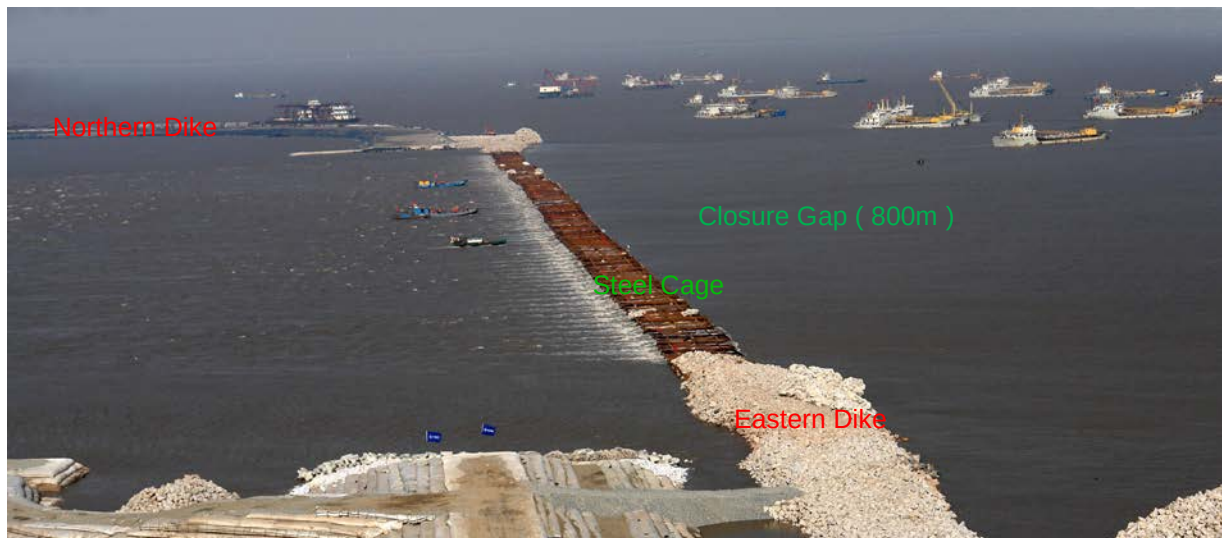
Figure 7. Closure gap after placement of steel cage.
