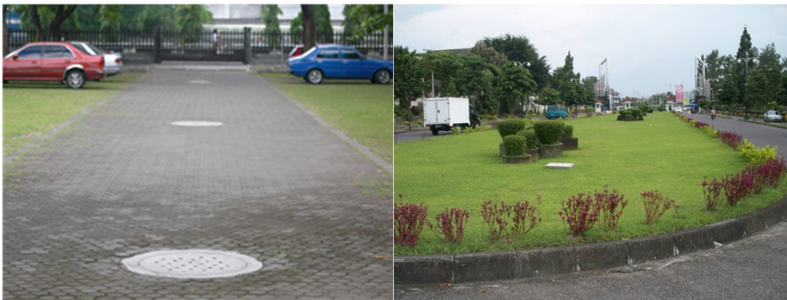
Figure 5. Recharge well and rain garden
