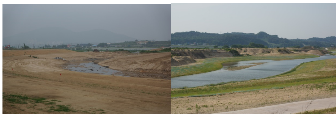
Figure 5. The old-channel restoration project (left: removing levee at upstream inlet, 2014; right: restoring the old channel, 2015)
