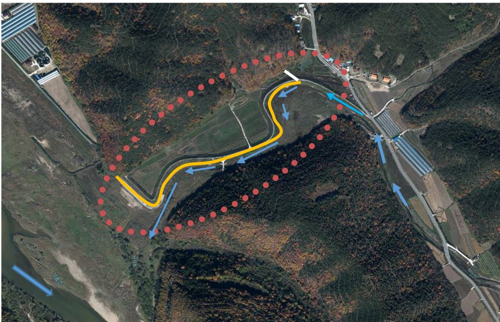
Figure 7. A sample site for the Case 2 for levee removal for increase in flood conveyance and floodplain restoration
