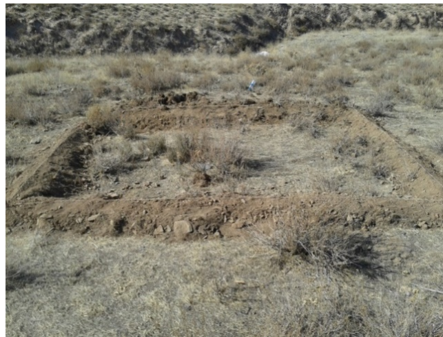
Figure 2. A view of the constructed Bankette structure.
