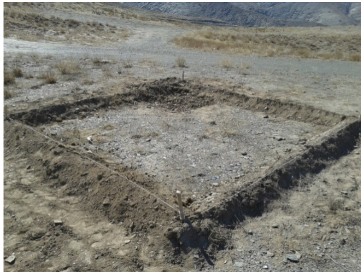
Figure 3. A view of the constructed Negarim Microcatchment.
