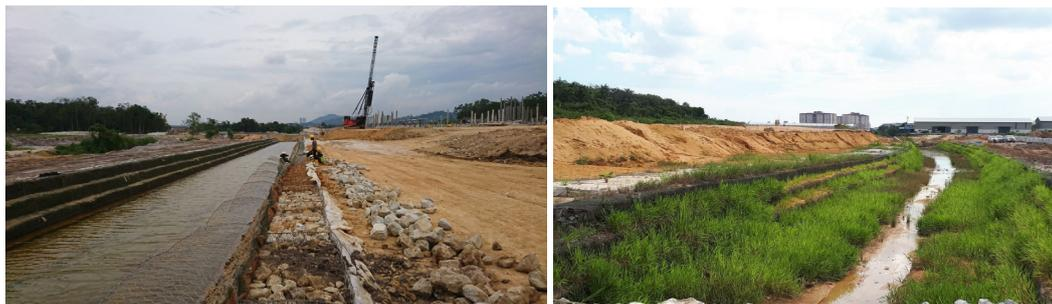
**Figure 10.** On going river rehabilitation work using bio-engineering technique.
