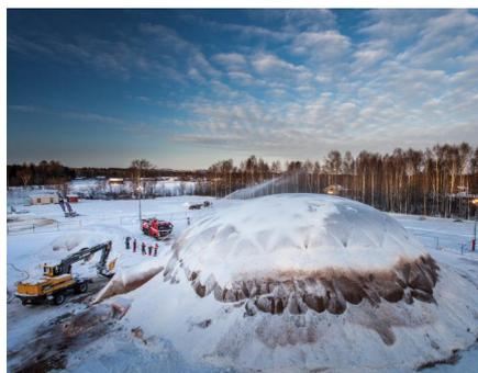
**Figure 5.** Pykrete Dome in Juuka, Finland, built with inflatable mould (Vasiliev and Pronk, 2015).
