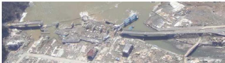
Figure 1. Washed away concrete girder bridge (Mazinani et al., 2014).
