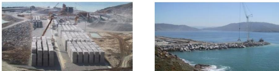
**Figure 12.** Block manufacturing yard and crane laying blocks.
