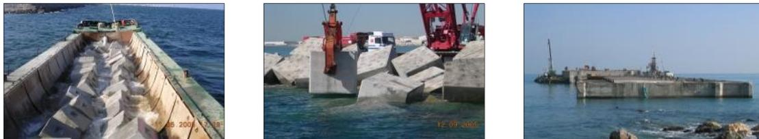
Figure 29. Construction stages. Dumping barge, crane blocks placement and caisson sinking.
