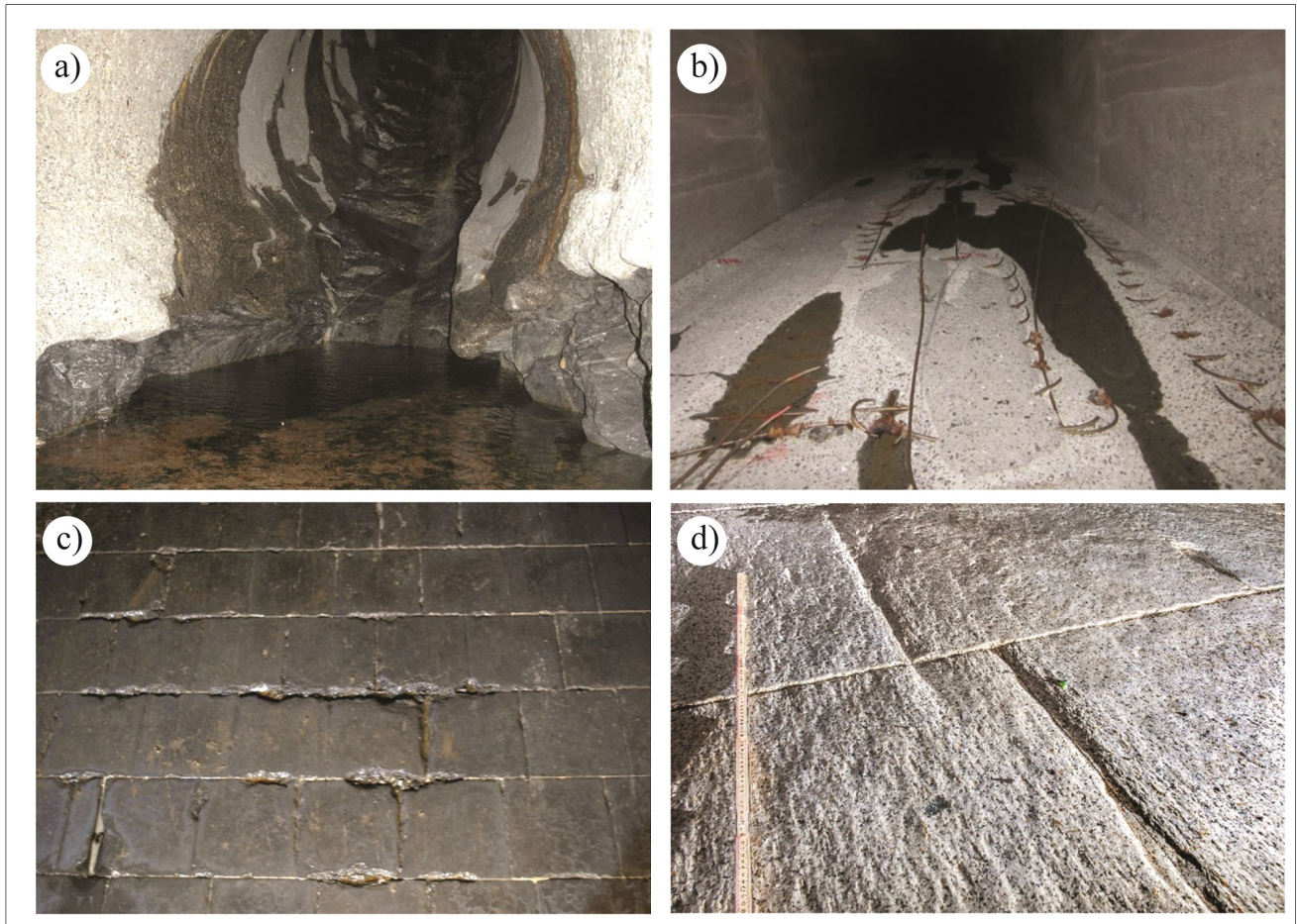
Figure 1. Hydroabrasion examples, a) abrasion at Val d'Ambra SBT (CH) into the concrete lining and rock underground (M. Müller-Hagmann), b) incision channels of the reinforced concrete lining of Asahi SBT (JP) (KEPCO, 2012), hydroabrasive damages at c) cast basalt tiles in Runchez SBT (CH) (M. Müller-Hagmann) and d) at the granite lining of Pfaffensprung SBT (CH) (VAW).
