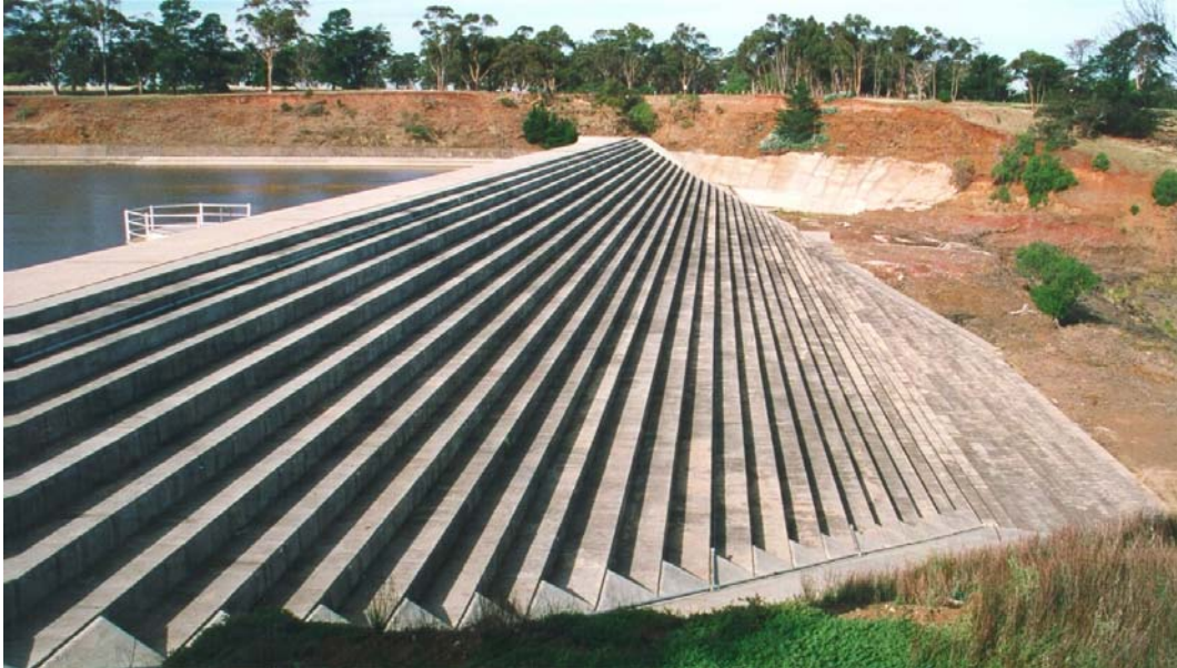
Fig. 3 - Melton dam stepped spillway on 30 January 2000 - Completed in 1916, the Melton dam was equipped in 1994 with a secondary stepped spillway ( Q_{des} = 2,800 \text{ m}^3/\text{s} , h = 0.6 \text{ m} )
