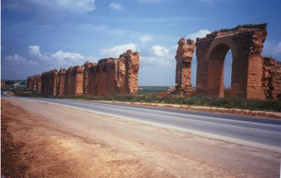
(B) Arcades at Oued Milliane, Carthage aqueduct, Tunisia on 3 April 2003 (Courtesy of Jean-Claude LITAUDON)
