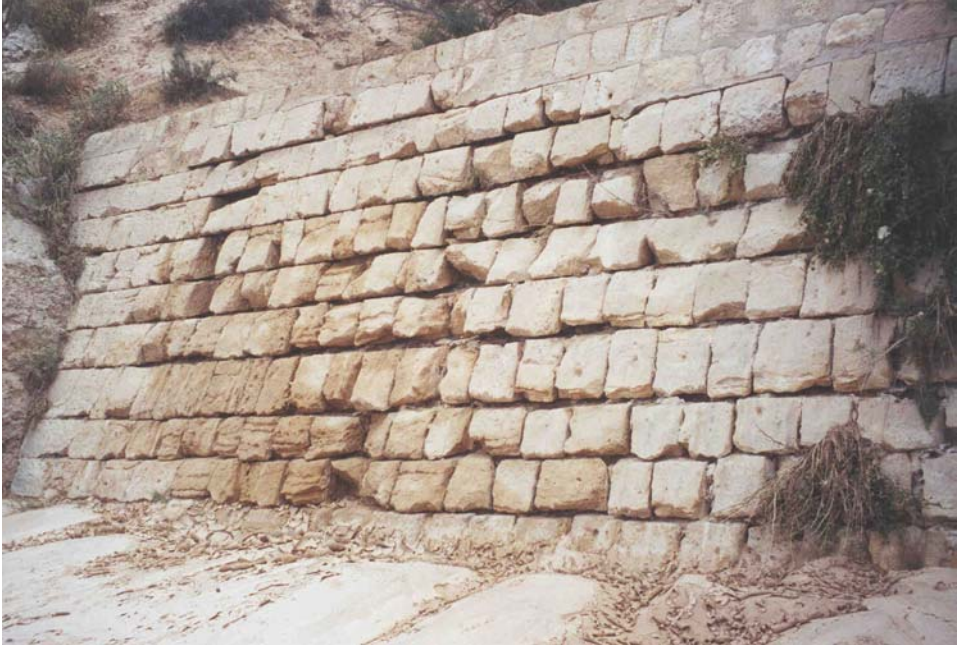
Fig. 1 - Ancient hydraulic works (A) Nabataean dam (1st century BC) on the Mamshit stream (also called Mampsis or Kunub) on 10 May 2001 (Courtesy of Dennis MURPHY) - Downstream slope of the dam wall
